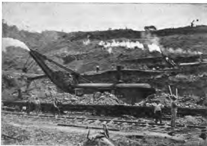
STEAM SHOVEL LOADING FLAT CARS.
